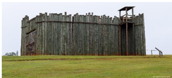
A portion of the Andersonville Prison showing its composition and proportions. This is the prison gate where incoming prisoners were processed. The highest structure in the corner (right) is a 'pigeon roost' guard post. (dp Sager Photography)
